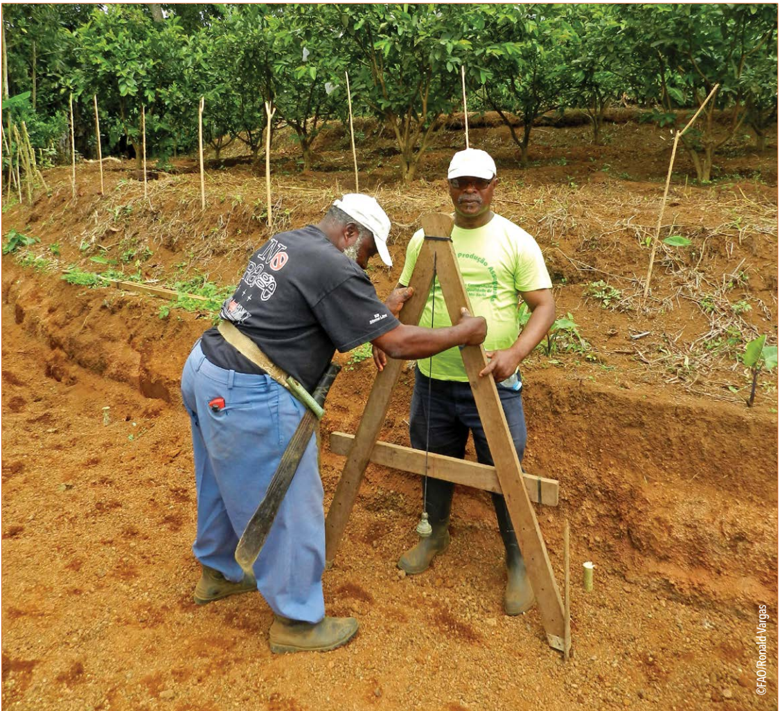
Figure 26: Terrace construction for erosion control in Sao Tome.
